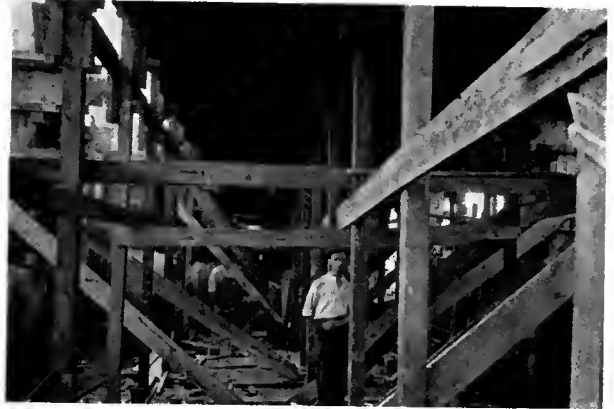
FIG. 3. VIEW UNDER SUPPORTS
